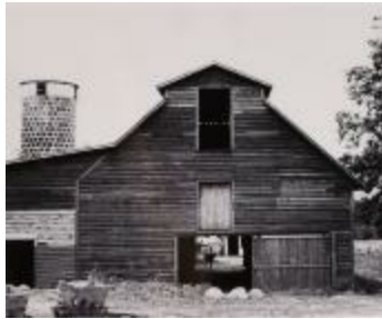
Barn and Silo with Cow in Doorway (2016.24.3)
