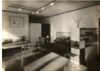
Masters' House Interior (2019.3.7)
