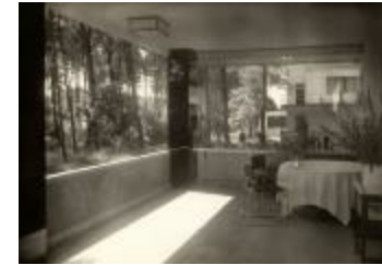
Masters' House Interior (2019.3.8)
