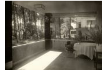
Masters' House Interior (2019.3.8)
