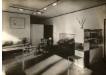
Masters' House Interior (2019.3.7)
