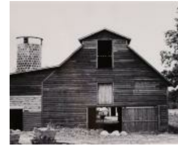
Barn and Silo with Cow in Doorway (2016.24.3)
