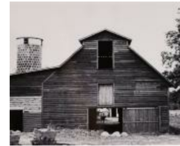
Barn and Silo with Cow in Doorway (2016.24.3)
