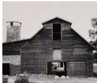
Barn and Silo with Cow in Doorway (2016.24.3)
