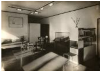
Masters' House Interior (2019.3.7)
