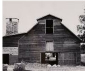
Barn and Silo with Cow in Doorway (2016.24.3)
