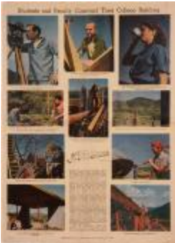
"Students and Faculty Construct their College Building" (1995.8.1)
