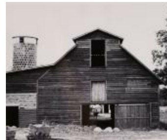
Barn and Silo with Cow in Doorway (2016.24.3)
