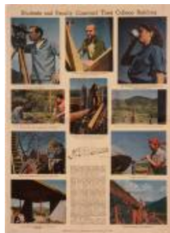
"Students and Faculty Construct their College Building" (1995.8.1)
