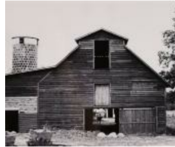
Barn and Silo with Cow in Doorway (2016.24.3)
