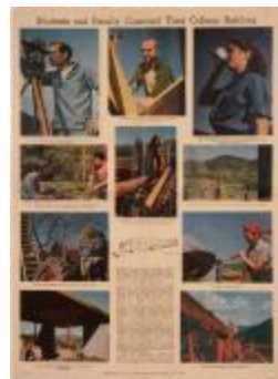
"Students and Faculty Construct their College Building" (1995.8.1)
