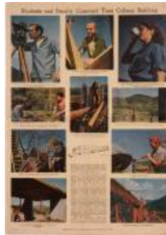
"Students and Faculty Construct their College Building" (1995.8.1)
