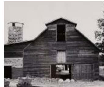
Barn and Silo with Cow in Doorway (2016.24.3)
