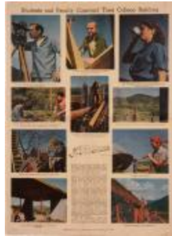
"Students and Faculty Construct their College Building" (1995.8.1)
