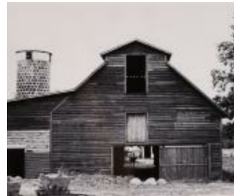
Barn and Silo with Cow in Doorway (2016.24.3)
