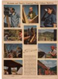
"Students and Faculty Construct their College Building" (1995.8.1)
