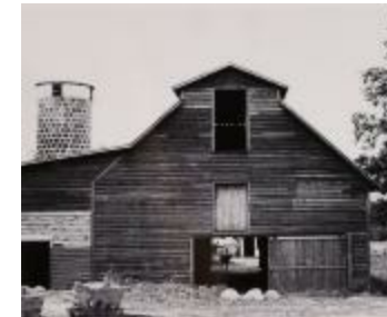
Barn and Silo with Cow in Doorway (2016.24.3)
