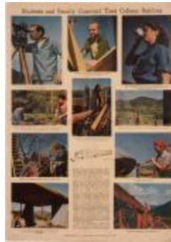
"Students and Faculty Construct their College Building" (1995.8.1)
