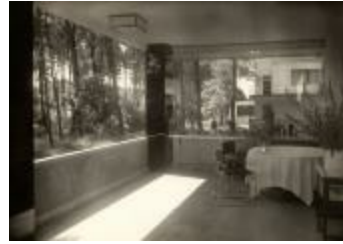
Masters' House Interior (2019.3.8)
