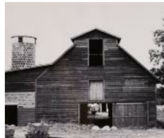
Barn and Silo with Cow in Doorway (2016.24.3)
