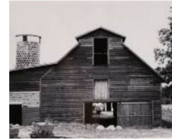
Barn and Silo with Cow in Doorway (2016.24.3)
