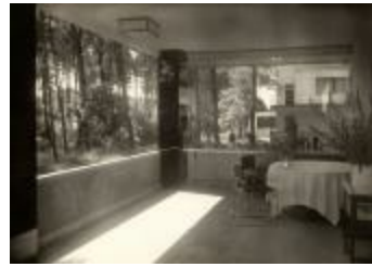
Masters' House Interior (2019.3.8)
