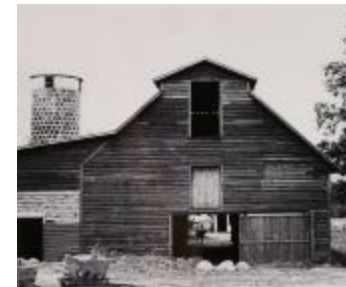
Barn and Silo with Cow in Doorway (2016.24.3)
