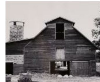
Barn and Silo with Cow in Doorway (2016.24.3)
