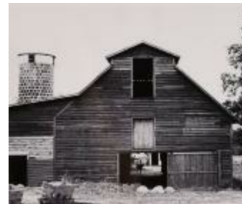
Barn and Silo with Cow in Doorway (2016.24.3)
