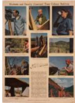
"Students and Faculty Construct their College Building" (1995.8.1)
