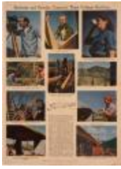
"Students and Faculty Construct their College Building" (1995.8.1)
