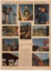
"Students and Faculty Construct their College Building" (1995.8.1)
