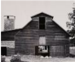
Barn and Silo with Cow in Doorway (2016.24.3)
