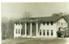
The back of the YMCA building (2003.7.7)
