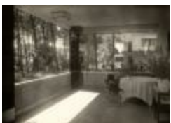
Masters' House Interior (2019.3.8)
