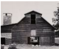
Barn and Silo with Cow in Doorway (2016.24.3)
