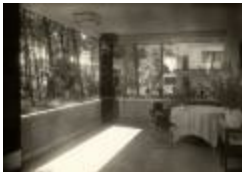
Masters' House Interior (2019.3.8)
