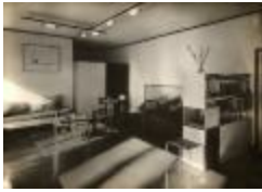
Masters' House Interior (2019.3.7)
