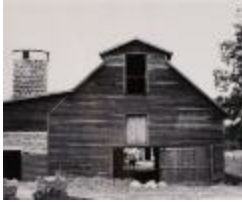
Barn and Silo with Cow in Doorway (2016.24.3)
