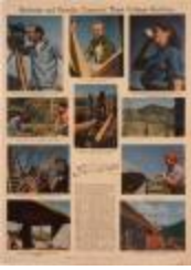
"Students and Faculty Construct their College Building" (1995.8.1)
