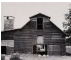
Barn and Silo with Cow in Doorway (2016.24.3)
