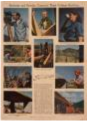
"Students and Faculty Construct their College Building" (1995.8.1)
