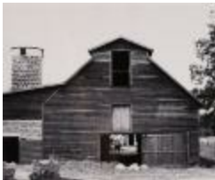
Barn and Silo with Cow in Doorway (2016.24.3)
