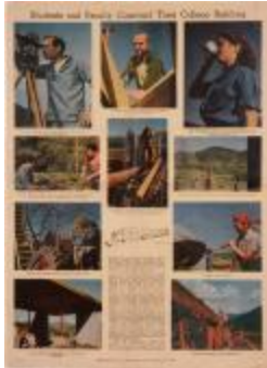
"Students and Faculty Construct their College Building" (1995.8.1)
