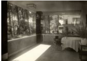
Masters' House Interior (2019.3.8)
