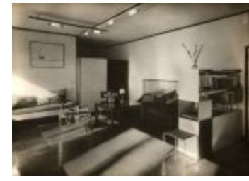
Masters' House Interior (2019.3.7)
