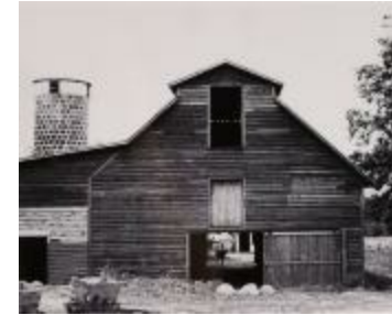
Barn and Silo with Cow in Doorway (2016.24.3)
