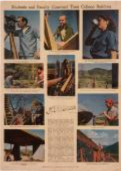
"Students and Faculty Construct their College Building" (1995.8.1)
