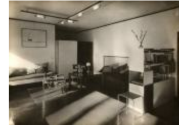
Masters' House Interior (2019.3.7)
