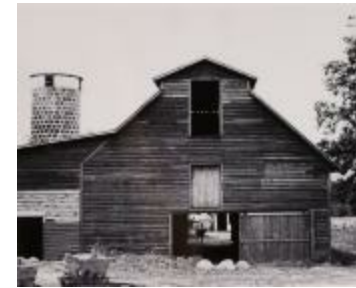
Barn and Silo with Cow in Doorway (2016.24.3)
