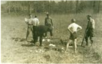
Black Mountain College Work Program at Blue Ridge Assembly (2003.7.1.22)
