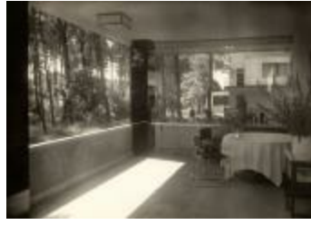
Masters' House Interior (2019.3.8)
