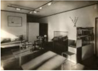
Masters' House Interior (2019.3.7)
