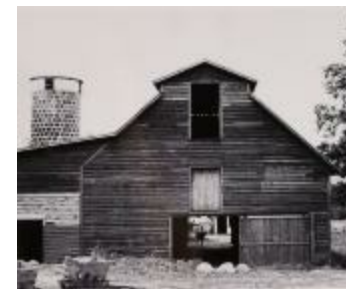
Barn and Silo with Cow in Doorway (2016.24.3)
