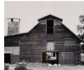
Barn and Silo with Cow in Doorway (2016.24.3)
