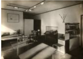
Masters' House Interior (2019.3.7)
